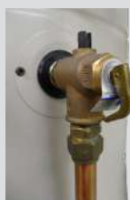
TPR position - top of cylinder
